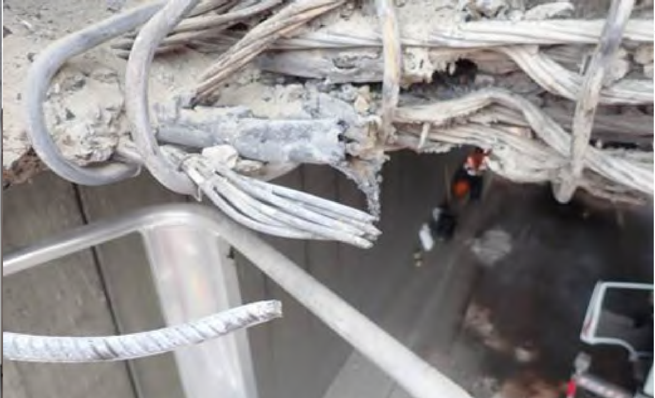
Split tendon in the bottom flange of the main beam
